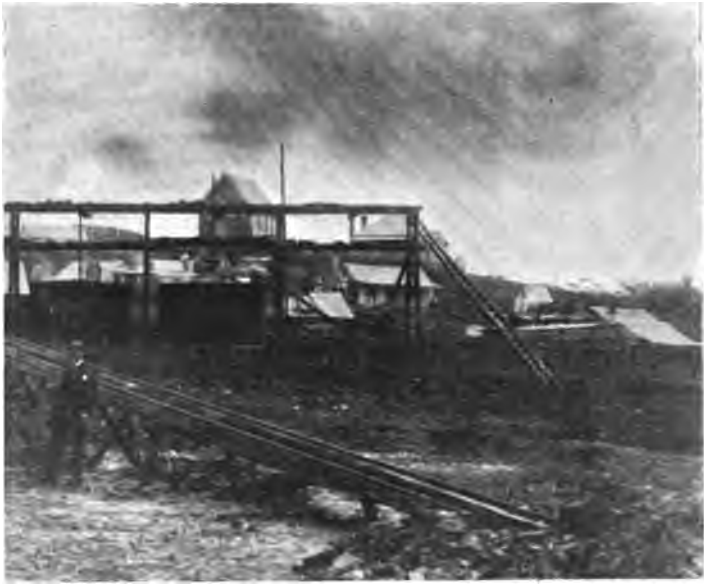
FIG. 149.—AGITATION TANKS.
